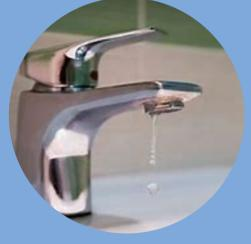
Check for leaky faucets! These leaks are usually obvious and a leaking faucet often just needs only a replacement part or new o-ring to be fixed.
