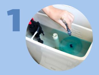
If you suspect a toilet leak, place a couple drops of food coloring in the tank and wait 15-30 minutes. If you see the colored water in the toilet bowl this is indicative of a worn toilet tank flapper.
